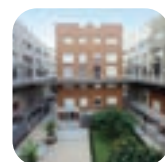
05 Town houses Schell Casas en condominio 2007
