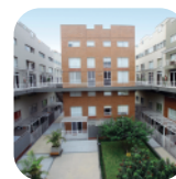
05 Town houses Schell Casas en condominio 2007
