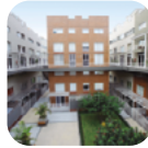
05 Town houses Schell Casas en condominio 2007
