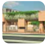
19 Veranda Piura Centro comercial 2015 – 2016
